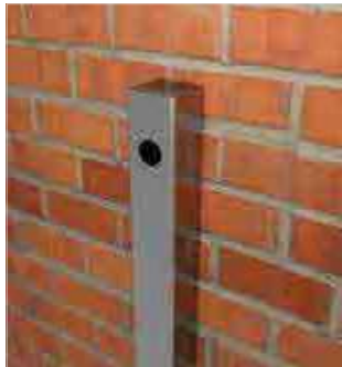
1 Drill a 25mm diameter hole through front wall of post
