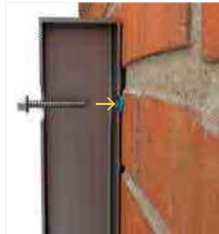
2 Drill rear wall of post with required diameter for fixing and then fix post to wall. Insert appropriate fixing into the wall for affixing post
