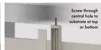
Screw top/bottom plate to centre support rail
