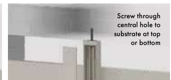
Screw top/bottom plate to centre support rail
